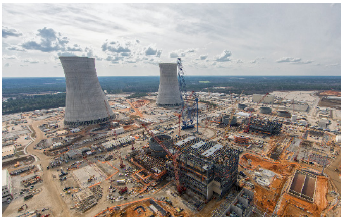
Plant Vogtle - Under Construction Photo Source: gpbnews.org
